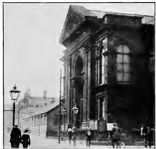
SLIDE No. 9.—MAWDSLEY STREET CONGREGATIONAL CHURCH.
